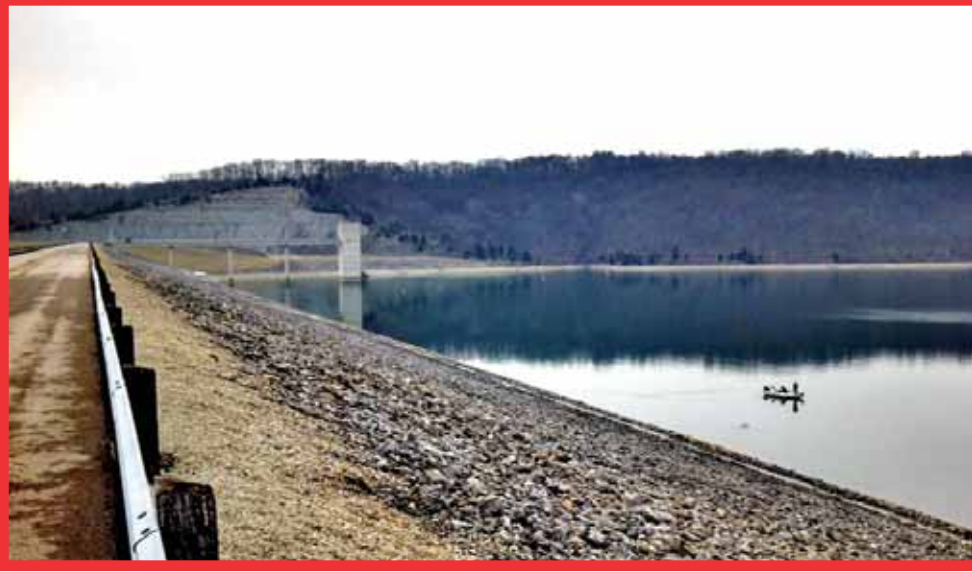
Left Photo: North side of Brookville Lake Dam on East Side. Rip Rap rock covers most of the North side of dam. Dam road closed to vehicles, foot traffic only allowed to cross dam. Right Photo: The Whitewater River north of SR 44 Bridge. Free parking and easy access to bank fishing on both north and south side of bridge. (Author Photos)
