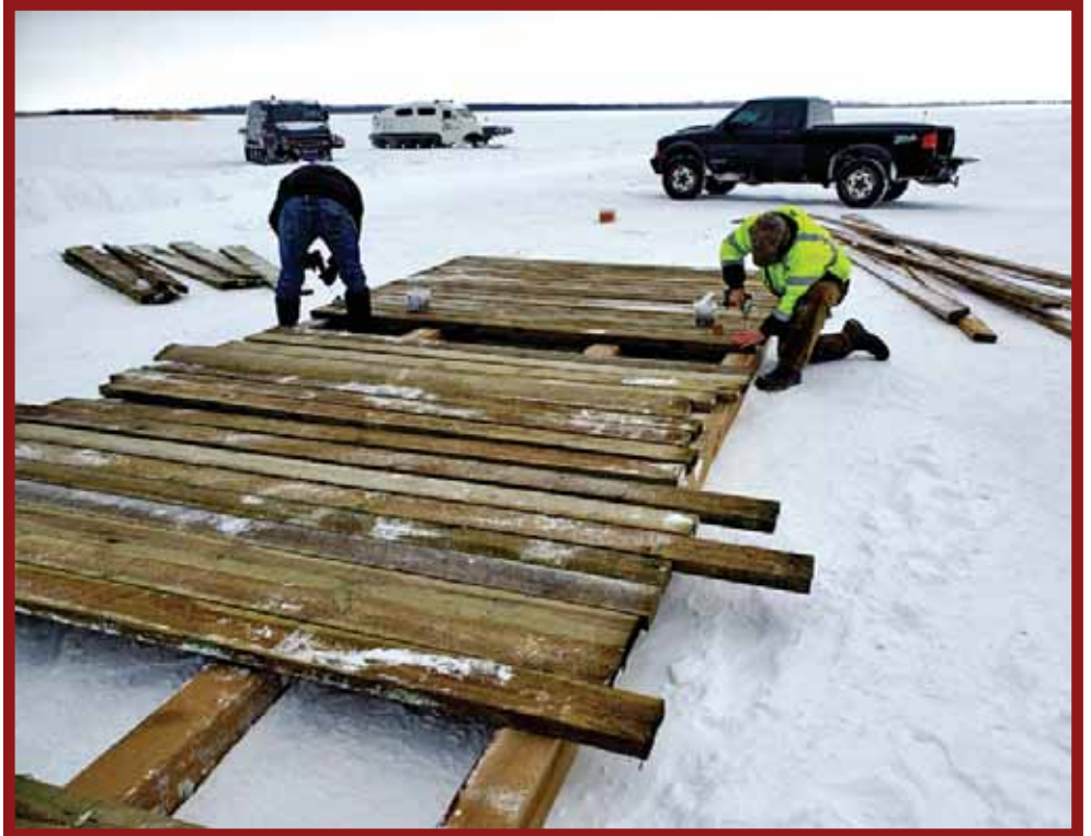
Resort owners building bridges across cracks in ice. (Photo by Joe Henry, LOW Tourism Bureau)
