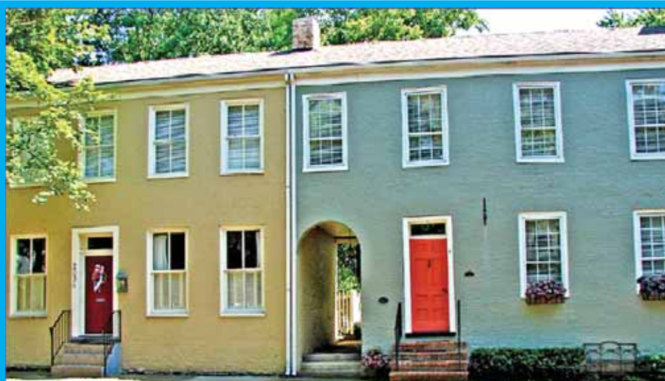
2 Shortridge Archway (2) located at 205 West Main St., c. 1820. (Author Photo)
