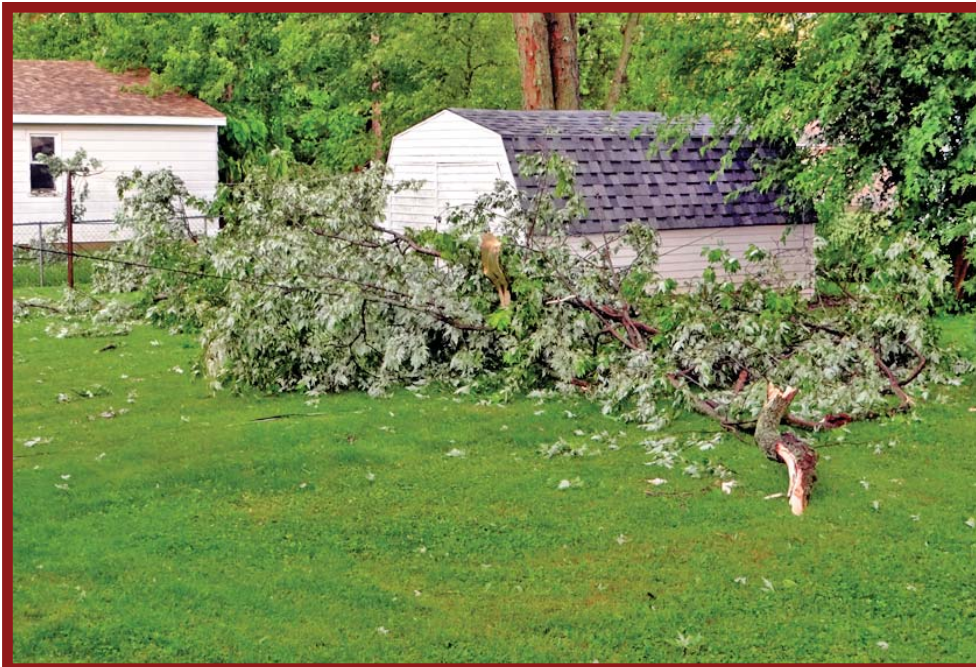
Storm damage behind 403 and 405 East School June 18, 2021. (Author Photo)
