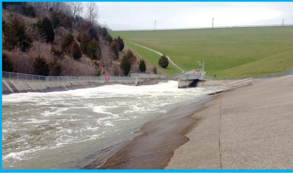
This is a photo of the stilling basin when the Corps of Engineers was utilizing their flood control method of releasing excess rain water from the lake. (Author Photo)
