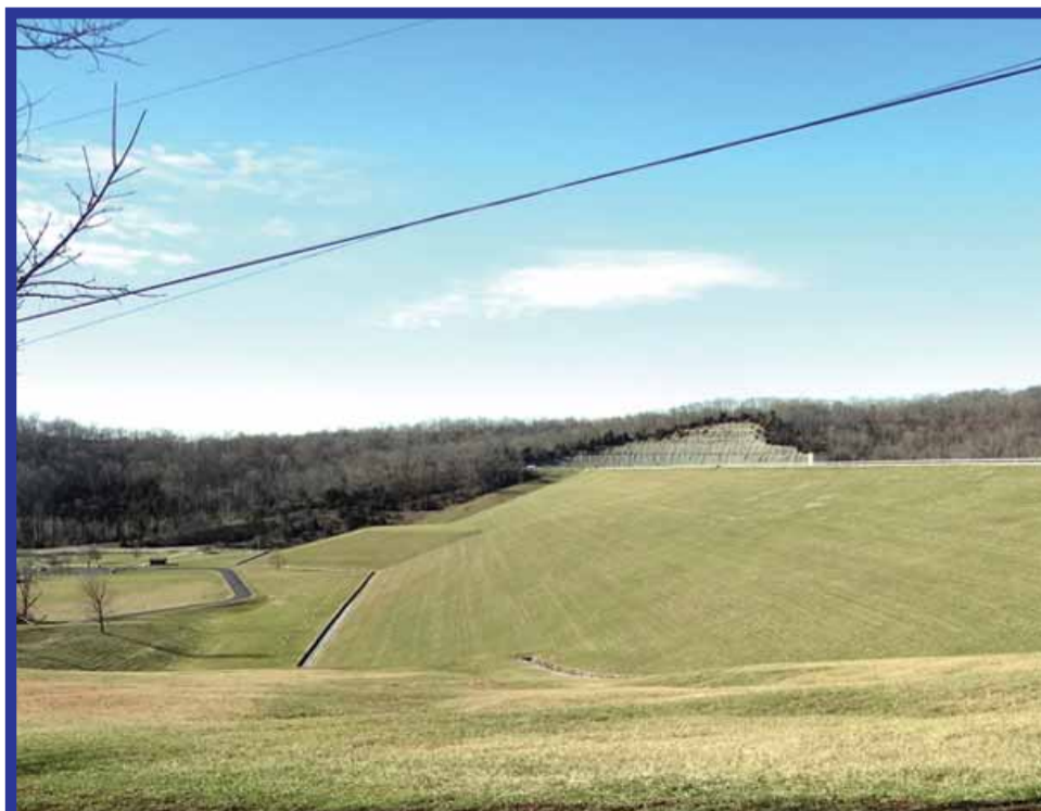
Brookville Lake Dam, photo taken January 7, 2020 looking west from east side dam access road and parking area. Good view of Cut-away for Spillway on far west end of dam, Stilling Basin mound, Parking and Tailwater Access from SR 101. (Photo by Ray Dickerson)
