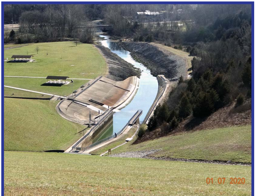
Stilling Basin looking down from the top of the Brookville Lake Dam. It was a beautiful day when I took this photo. Notice the three fisher persons trying their luck at the railing. I walked across the dam enjoying the nice sunny day. (Photo by Ray Dickerson)
