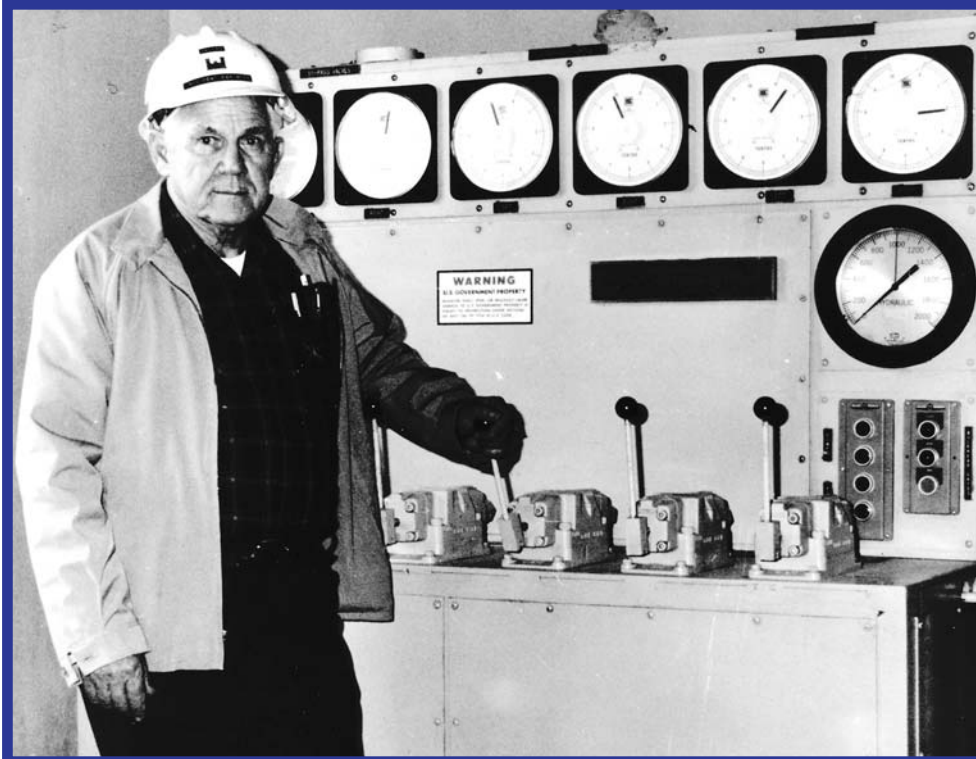
C.J. Walter, Brookville Lake Resident Engineer, January 24, 1974 standing at the Control Valves, which had been activated earlier that day closing the Dam gates to hold back the East Fork of the Whitewater River, which began filling the Valley with water.
