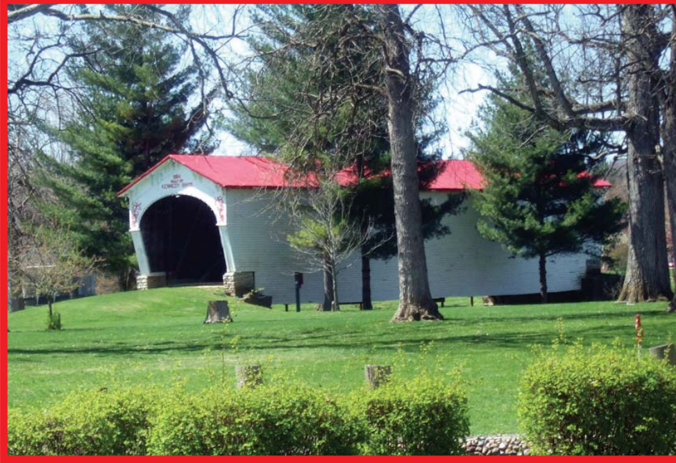
Kennedy Bridge located in Roberts Park in Connersville, Indiana.
