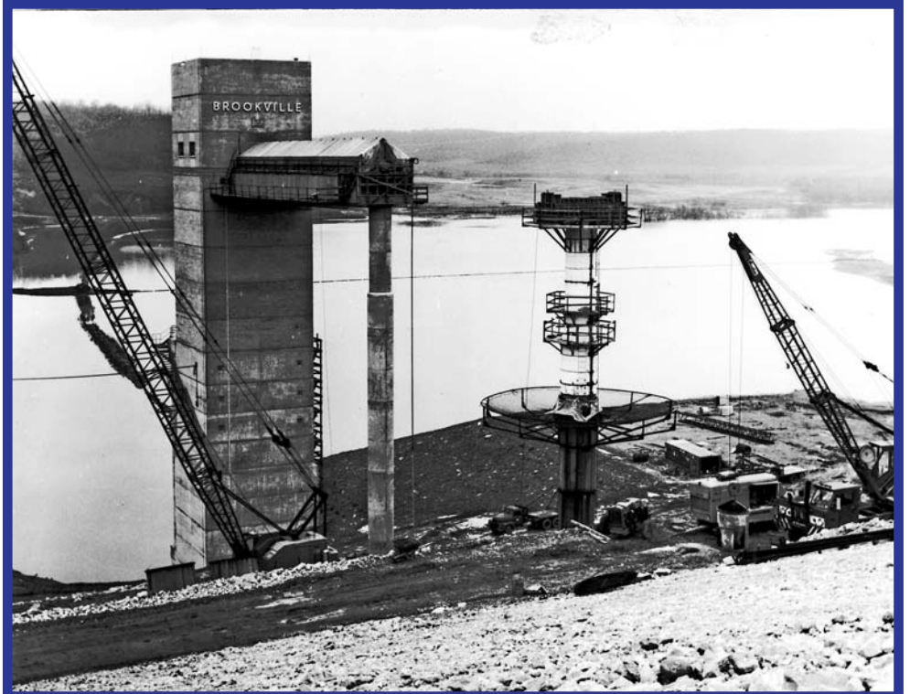
Tower access construction underway. C.J. Walter took me down the dam to access the tower on 1-24-74. The dam was covered with mud and clay (see story). The return trip up the dam took C.J. a 3rd time before making it all the way to the top and staying there.
