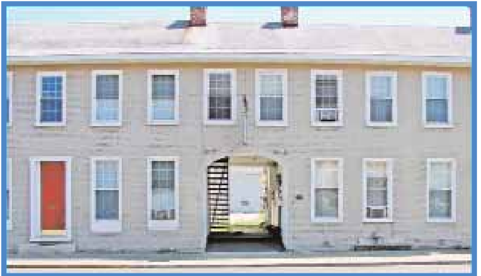
Backenstoers Archway (3) located at 139 East Main St., c. 1835. (Author Photo)
