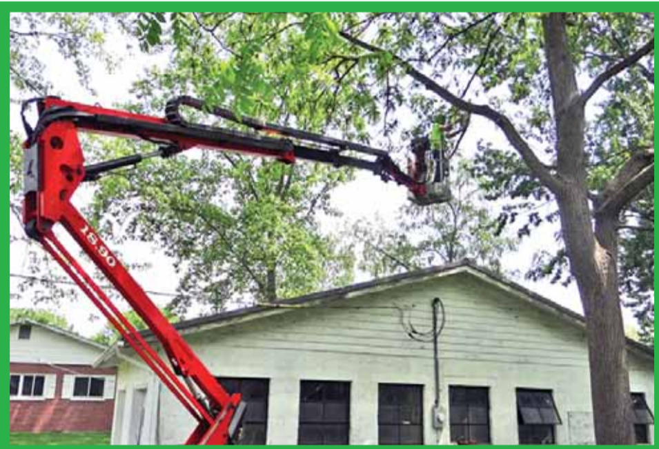
Jack trimming limbs back from neighbors building.
