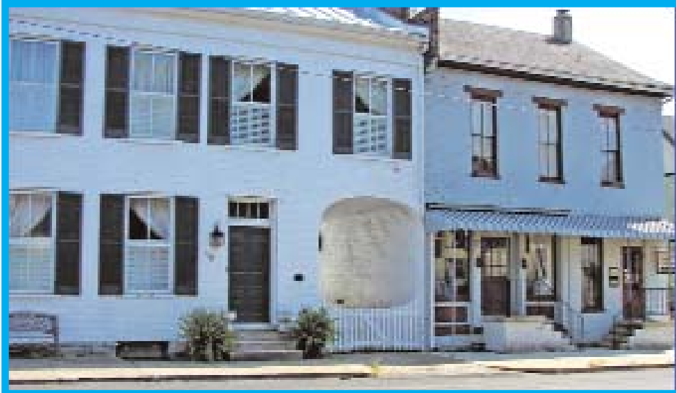
Malone Archway (3) located at 11 West Main St., c. 1836. (Author Photo)
