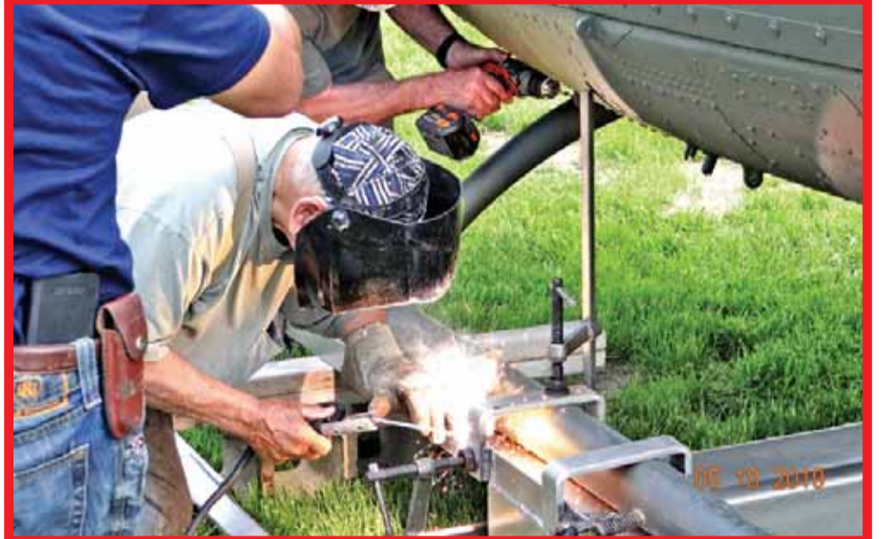
Left Photo: The Crane operator gently lowers the helicopter down to within inches of the aerial platform Joe Goebel built. Crane crew members align it up with the platform and motion for it to be placed on the platform. Right Photo: Once the helicopter is in place on the platform, Joe Goebel begins welding the first of four sets metal supports which will hold the Huey UH-569 and platform together as one unit. Other workers work in unison with Joe performing other tasks in the same vicinity.
