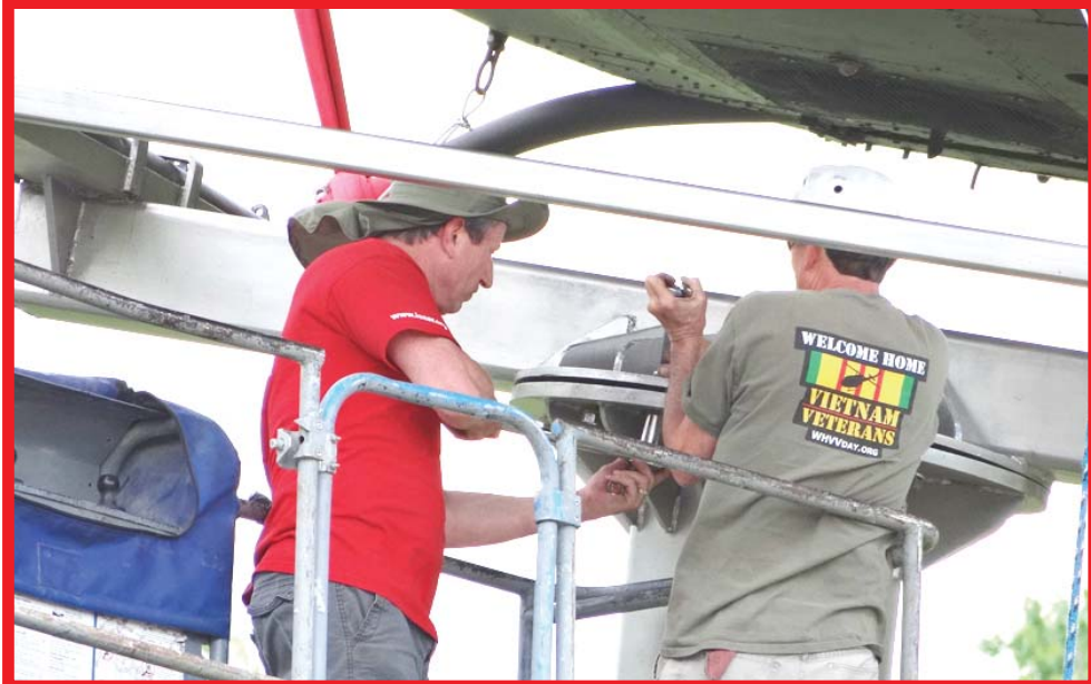
Left Photo: Charlie Walker and one of his crew tighten huge nuts and bolts that will hold the Huey and its aerial platform tightly together on the angled landing position. Right Photo: I took this picture at the Wayne County Veterans Memorial Park on June 4, 2019. It took a lot of hard work to put the Huey up on the tower, but its' home now!
