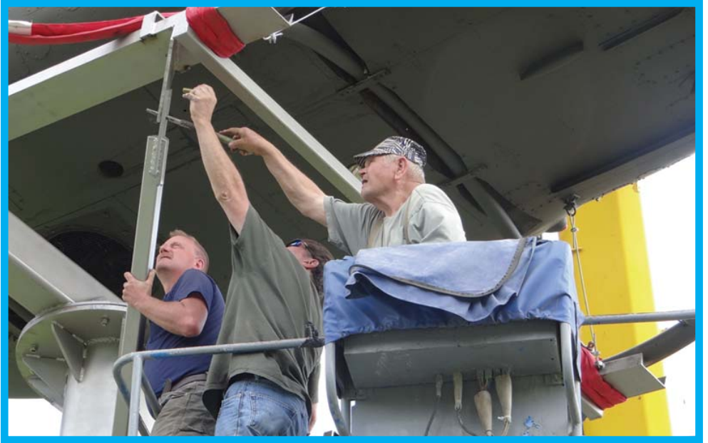
Left Photo: Beard Masonry of Richmond, IN (PH 765-969-0630) donated the use of this lift to secure Huey UH-569 to its tower (see right photo). Right Photo: Micah Clopper (C&C Crane Co) holds tower support in place while Joe Goebel aligns two connections with metal rod, while third guy inserts bolt in the other hole.
