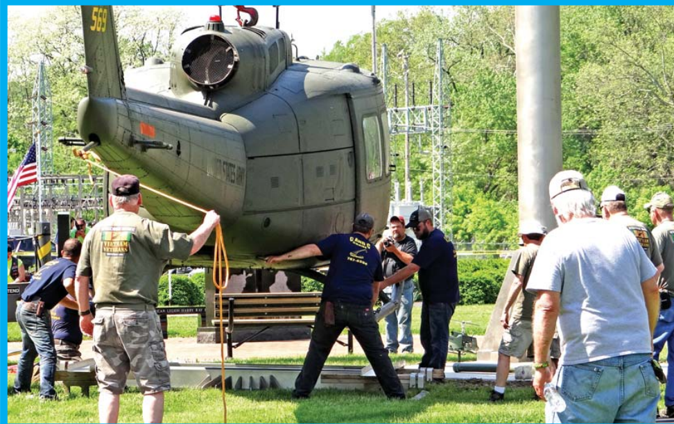
Left Photo: The Crane operator gently lowers the helicopter down to within inches of the aerial platform Joe Goebel built. Crane crew members align it up with the platform and motion for it to be placed on the platform. Right Photo: Once the helicopter is in place on the platform, Joe Goebel begins welding the first of four sets metal supports which will hold the Huey UH-569 and platform together as one unit. Other workers work in unison with Joe performing other tasks in the same vicinity.
