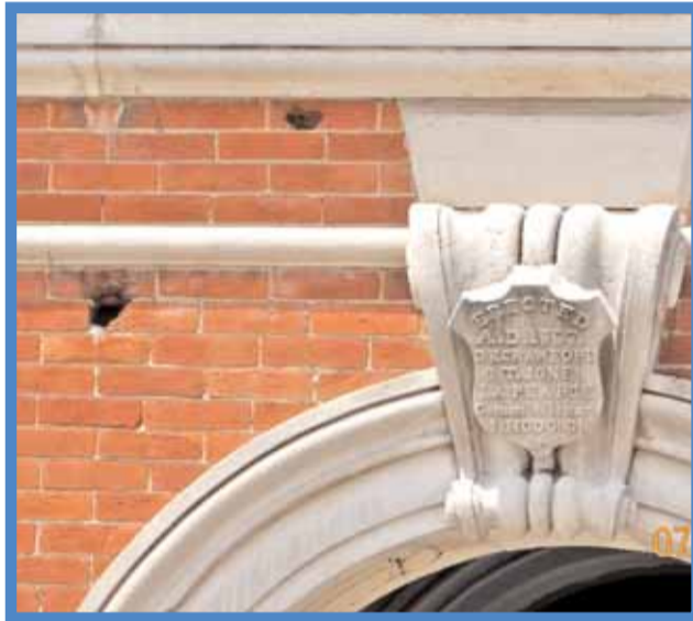
On August 13, 1873 Centerville citizens fired a cannon at this building knocking the Jail door off its hinges and left these holes you can still see today, 146 years later.
