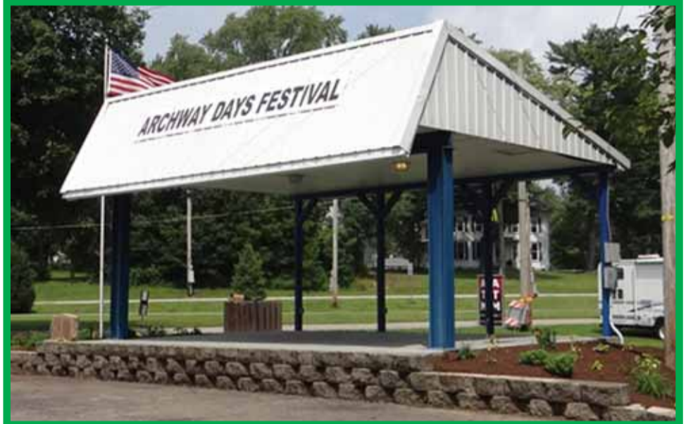
Maplewood Park Performance Center.
