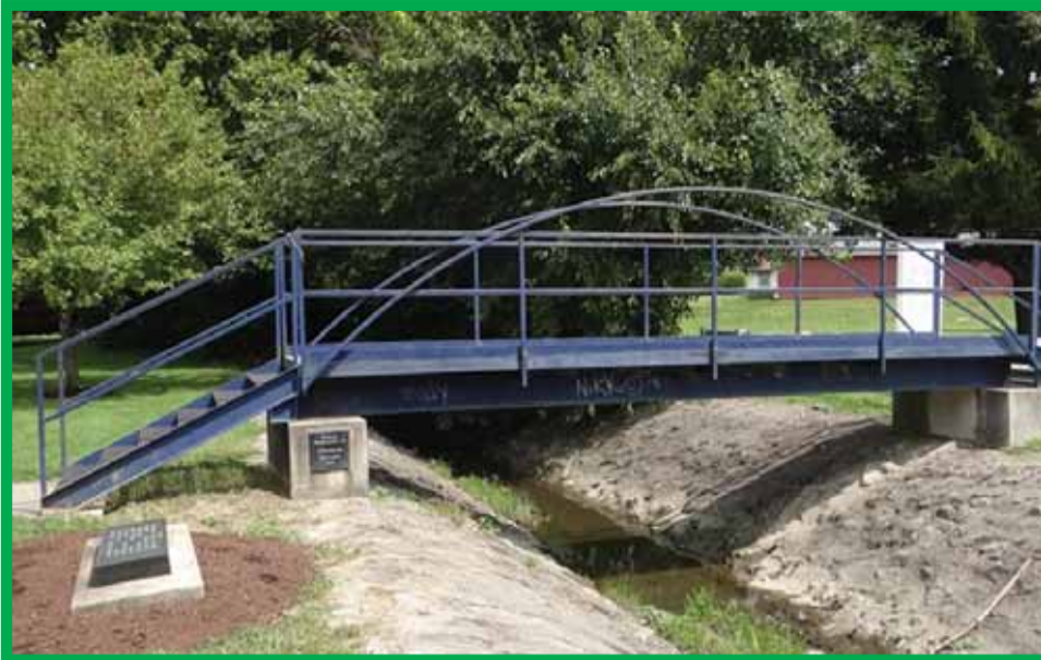
New Paddy's Run Bridge built after former bridge was washed away in flood.
