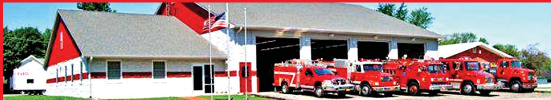
EVERTON'S NEW VOLUNTEER FIRE DEPARTMENT BUILDING AND THEIR FIVE FIRE TRUCKS
