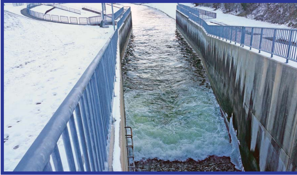
Bottom Right: Dam Stilling basin. (Author Photo)
