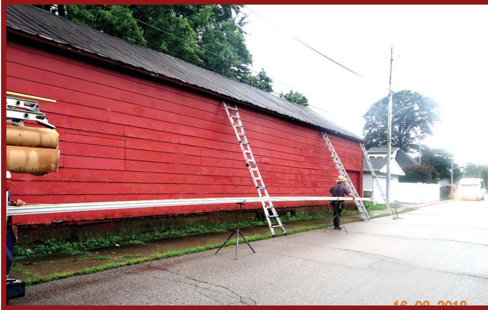
Left Photo: Kevin Sheets from JR'S Gutter Service runs out the continuous gutter from the back of their truck while Emanuel Fishers guides it to the end of the barn. Right Photo: I took this photo today November 10, 2018, showing the completed gutter work including leaf guard which they came back and added to the gutters on October 15, 2018. As you can see they did a really good job. When we got that day after day rain a week or so ago, no flooding, what a relief! (Author Photos)
