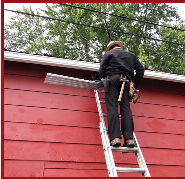
Left Photo: Kevin Sheets climbing ladder to finish attaching the straps that hold the gutter to the barn on north side of barn. Middle Photo: Emanuel Fishers preparing a leaf guard section which will be attached to the previous placed gutter to let the water run through and keep the leaves out. They work too! Right Photo: JR's Gutter Service truck. Contact JR's Gutter Service, Continuous Aluminum, Box 302, Fountain City, IN 47341, Ph: 765-847-2298. (Author Photos)
