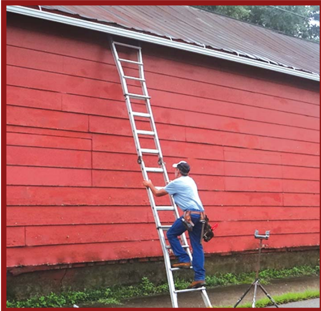
Left Photo: Kevin Sheets climbing ladder to finish attaching the straps that hold the gutter to the barn on north side of barn. Middle Photo: Emanuel Fishers preparing a leaf guard section which will be attached to the previous placed gutter to let the water run through and keep the leaves out. They work too! Right Photo: JR's Gutter Service truck. Contact JR's Gutter Service, Continuous Aluminum, Box 302, Fountain City, IN 47341, Ph: 765-847-2298. (Author Photos)
