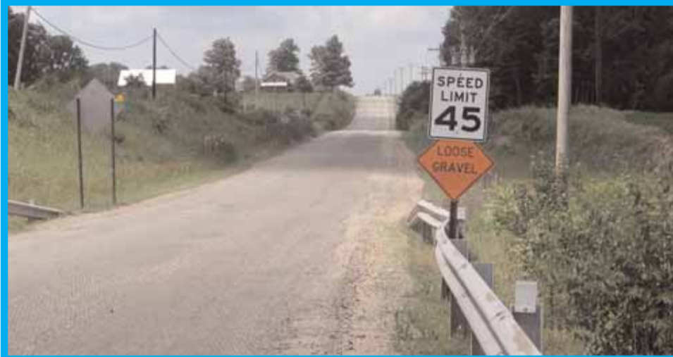
I took this photo on July 10th as you can see the road is very rough and loose gravel can be seen as well. I got quite a bit upset when I was told by a county official earlier in Liberty that day, that it might be several weeks before it was paved.
