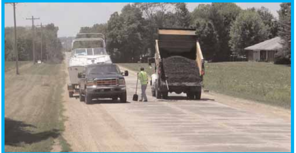
As I was on my way back to checking with my advertisers I stopped to take this photo of a Union County highway worker patching holes on Old SR 101. A glint of hope surfaced in my mind. They have to patch holes before paving. Hmmm!
