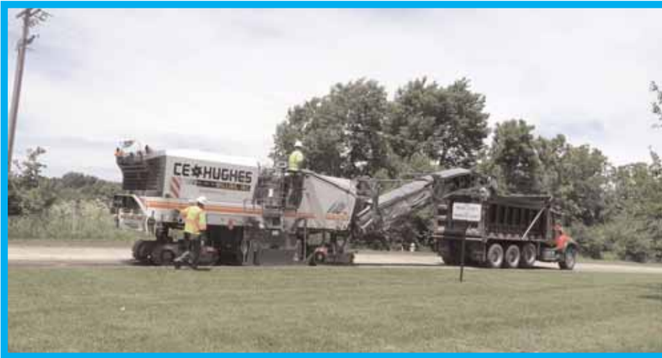
O'Mara Highway Construction crew grinding away top layer of Old SR 101 on June 5, 2018. Union County acquired this portion of Old SR 101 from the State of Indiana in 1973 when new SR 101 was built east of the new Brookville Lake dam.
