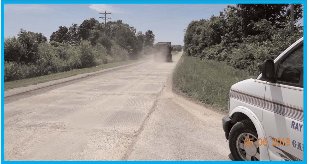
I took several photos of O'Mara's crews removing the top layer of Old SR 101 June 5th. I was told the last time it was resurfaced was in 1973. Since that time I've only saw Union County Highway workers patching old SR 101 like the photo below.
