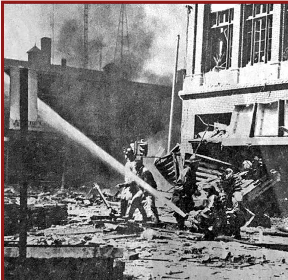
Richmond Fire fighters in middle of Main Street in front of Marting Arms Sporting Goods Store. Behind them is a car that was thrown into front window of Bartel's Department Store by the second explosion. (Palladium-Itemclipping submitted by Jack Bales)
