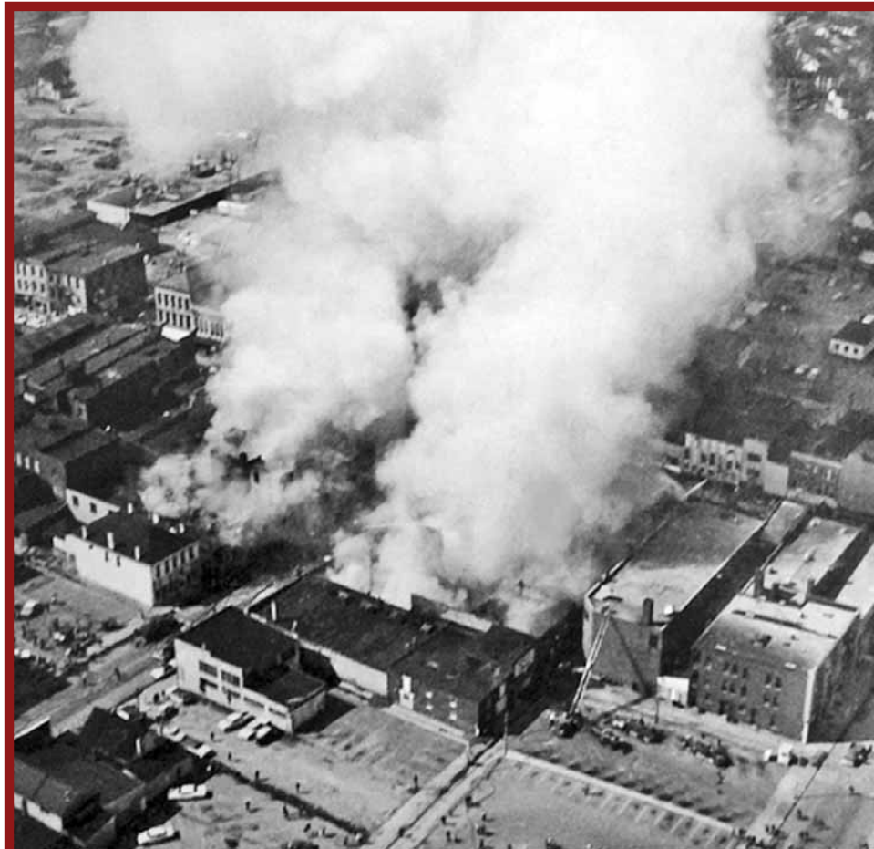
The afternoon of April 6, 1968. Two natural gas explosions level Vigran's Variety Store and Marting Arms Sporting Goods Store, fire consumes adjoining buildings in downtown Richmond, Indiana. Forty-one dead and 150 injured. (File Photo)
