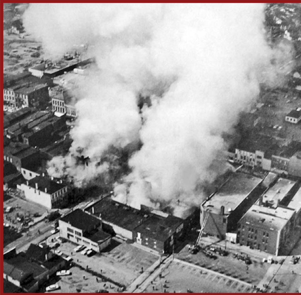
The afternoon of April 6, 1968. Two natural gas explosions level Vigran's Variety Store and Marting Arms Sporting Goods Store, fire consumes adjoining buildings in downtown Richmond, Indiana. Forty-one dead and 150 injured. (File Photo)
