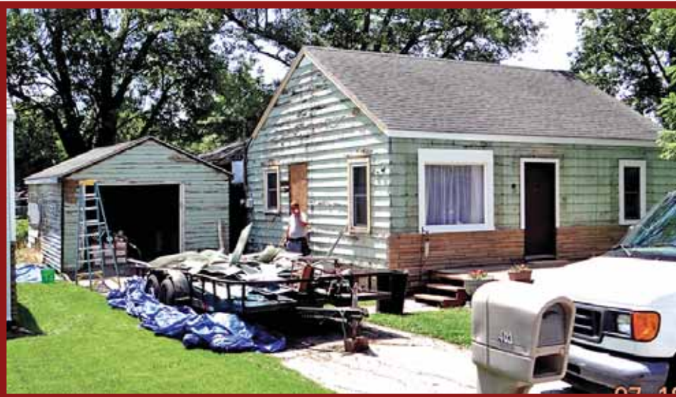
Our next phase began early in July 2016. James and Jennifer Bullen, owners of Bullen Roofing & Construction began removing siding and loading it on a trailer.
