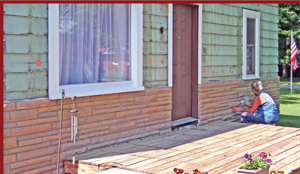
Here Jennifer is meticulously cleaning the rock facing with a brush. She spent an enormous amount of time carefully brushing the wall and power washed it clean on 7-19-2016.
