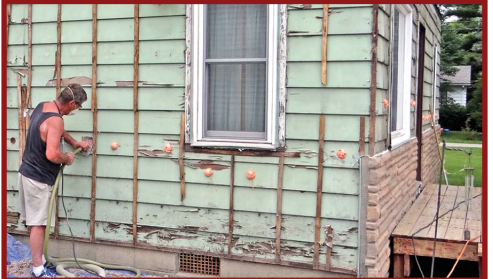
Here James Bullen is dense packing our walls with blown in insulation on July 12, 2016. James and Jennifer did their work in one of the hottest July's I can remember.
