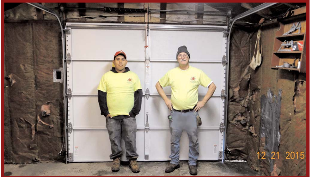
First phase of fixing up the home place was having Richmond's Complete Home Improvement & Overhead Door Co. install a brand new garage door on 12-21-2015.
