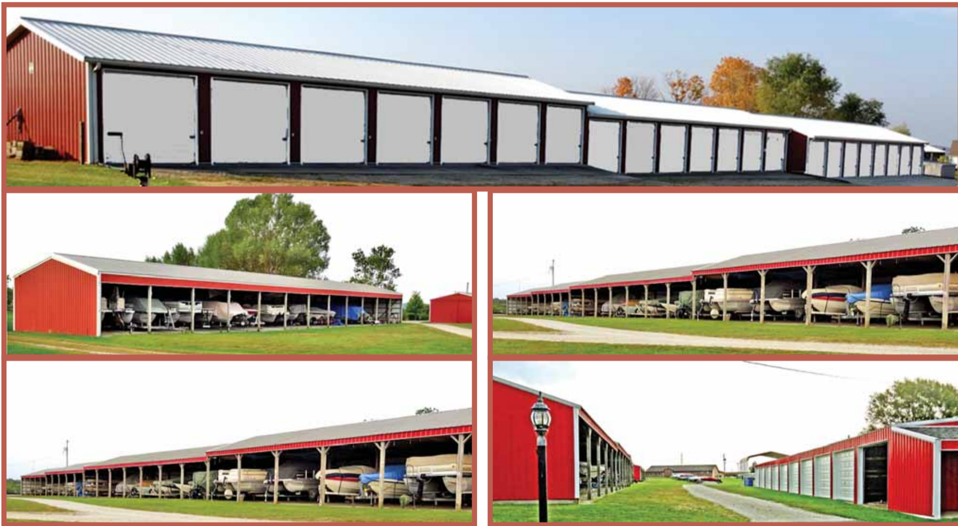
See Aerial view above and read article for information pertaining to Storage Units pictured above.
