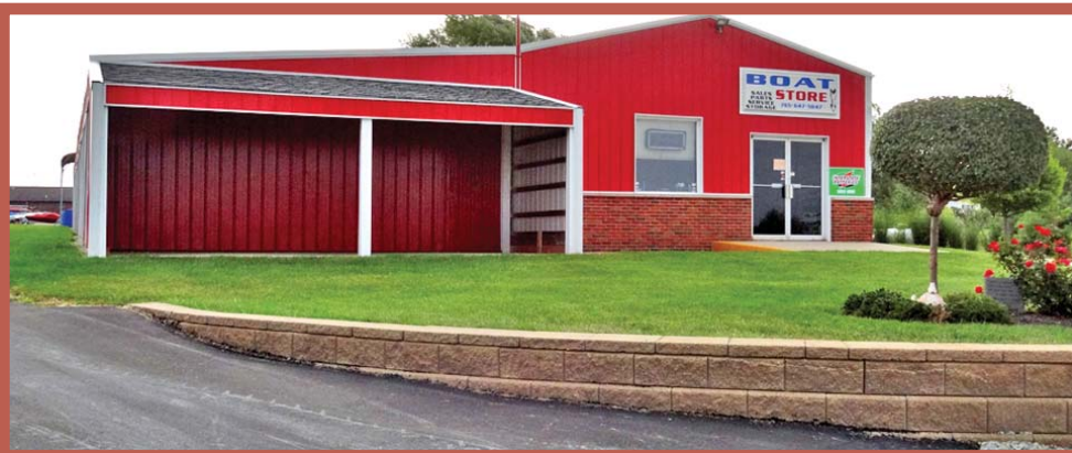
The retail location is in the west end of 1991 storage building, the rest of the building houses storage for boat parts, lawn equipment, tools and a maintenance shop.
