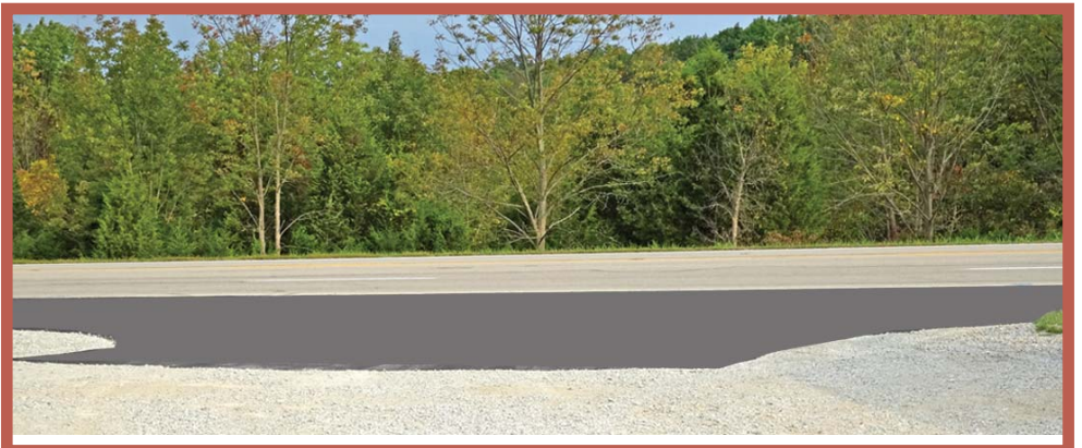
A new renovation is this paved driveway entrance off SR 101.
