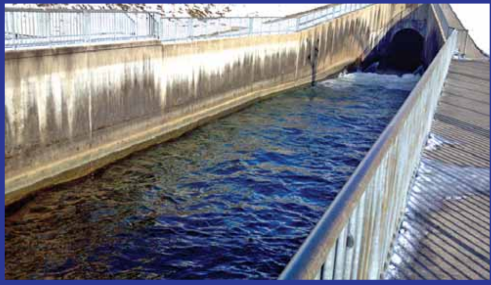
Top Left: As the water rushes thru the dam from the lake it empties into the Stilling Basin. The basin is a deep box like structure that calms and slows the water down before it enters the tailwater. Top Right: This photo is of the East Fork of the Whitewater River where SR 44 crosses it above Brookville Lake. Bottom Right: I caught this walleye in the winter on this jigging Rapala lure in Brookville Lake. (Author Photo)
