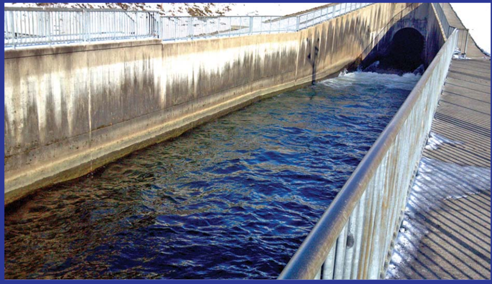
Top Left: As the water rushes thru the dam from the lake it empties into the Stilling Basin. The basin is a deep box like structure that calms and slows the water down before it enters the tailwater. Top Right: This photo is of the East Fork of the Whitewater River where SR 44 crosses it above Brookville Lake. Bottom Right: I caught this walleye in the winter on this jiggging Rapala lure in Brookville Lake. (Author Photo)
