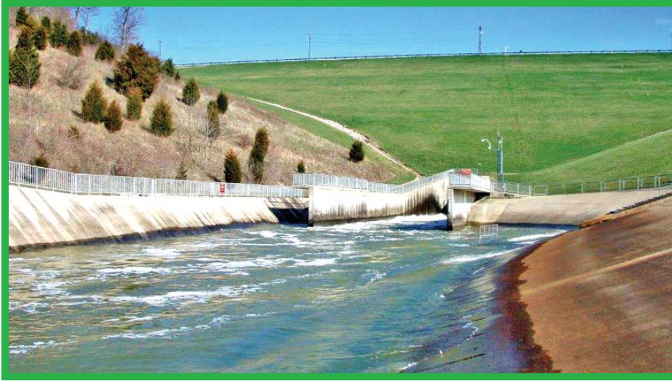
Left Photo: Stilling Basin below Brookville Lake Dam. Right Photo: Treaty Line Fisherman's Access Ramp on East Fork of Whitewater River. Bottom Right Photo: Brookville Lake Control Tower gates that control flow of water from Lake. (Author Photos)
