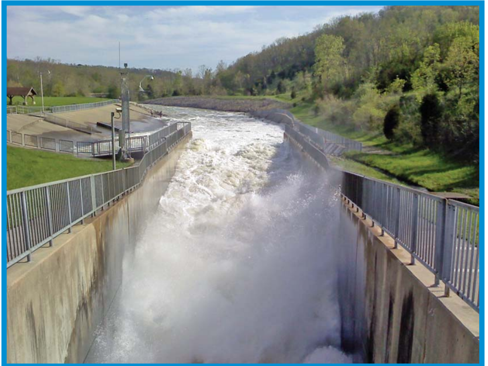
This picture shows how the stilling basin slows the flow of water down before leaving the stilling basin to continue on down the river. The water flow coming out of the lake in this picture is extremely high.. (Author Photo)
