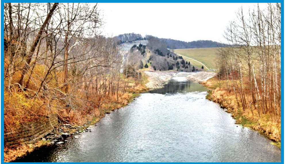
This is a picture of the tailwater (East Fork of Whitewater River) looking up towards the stilling basin from State Road 101 bridge. (Author Photo)
