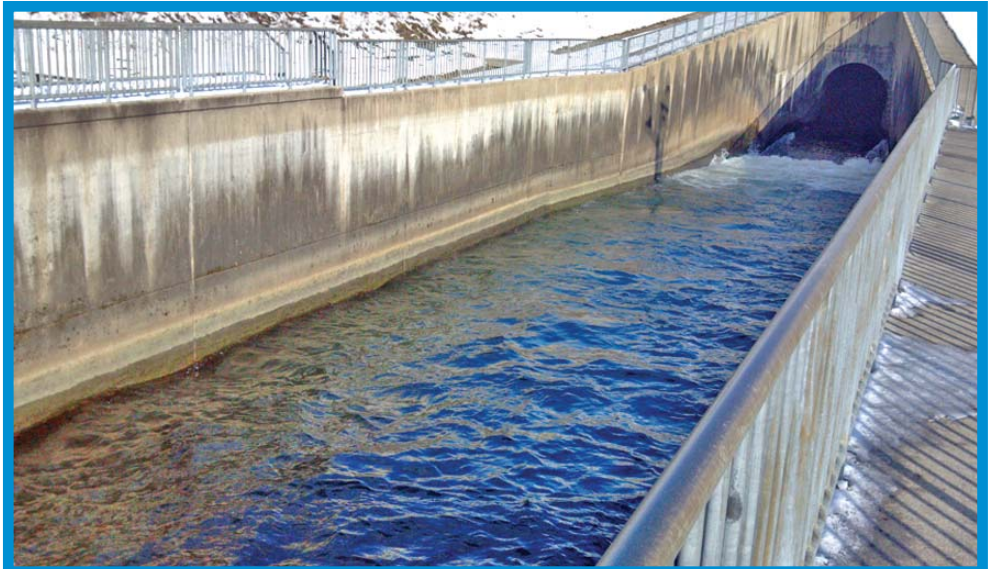
This is the stilling basin below the dam it is the 35 foot deep box I talk about in this article. (Author Photo)
