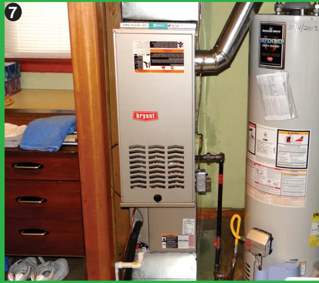
Old furnace and A/C removed 7-30, floor fixed 7-31, new furnace & A/C installed 8-1-14. All done in 3 days, wow! CONTINUED ON PAGE 30
