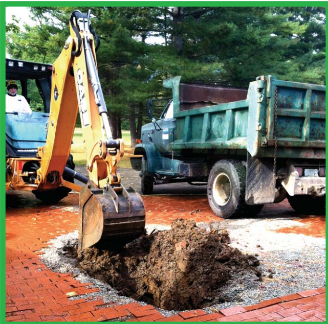
Veteran Inspired Memorial foundation footer being dug in front of Whitewater Memorial State Park office. Construction was paid for using donated funds. (Photo by Karen Schube)
