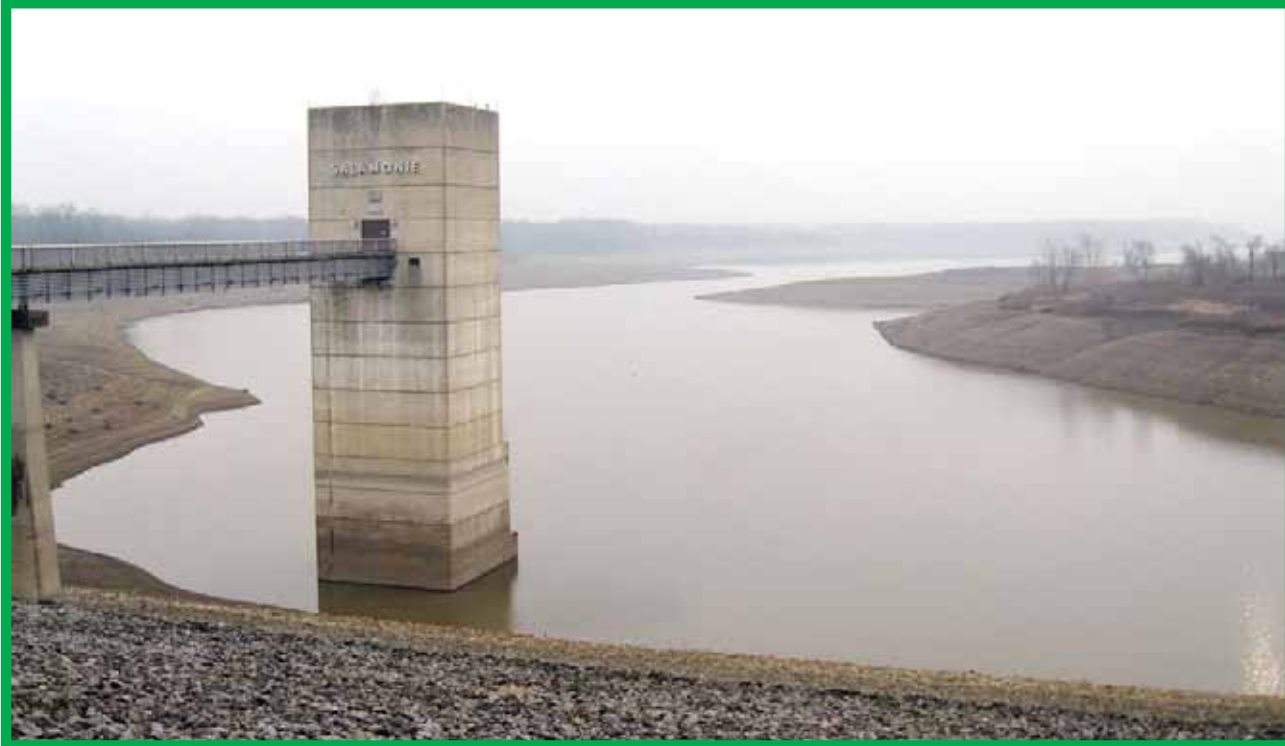
This is a photo taken from the Salamonie Dam overlooking the lake. The water is actually 4 feet below winter pool to allow for work at the Dora Boat Ramp being done to remove silt that had built up at the bottom of the ramp and allow it to continue to be accessible year round. (Photo by Author)
