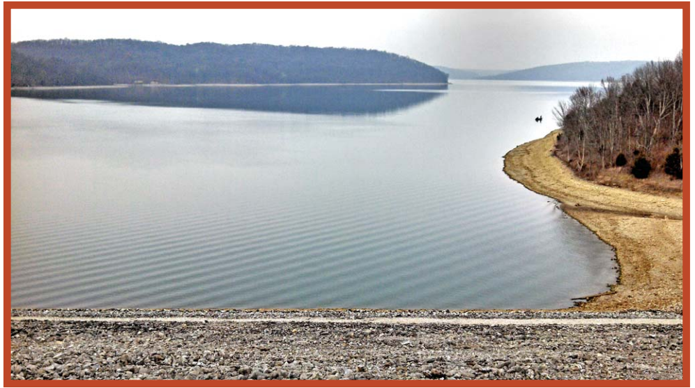
Brookville Lake Dam area looking north. Lake is at winter pool. (Author Photo)
