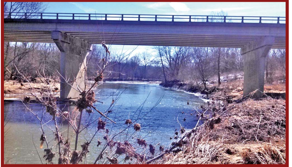
East Fork of Whitewater River above Lake flowing south under SR44 Bridge. (Author Photo)
