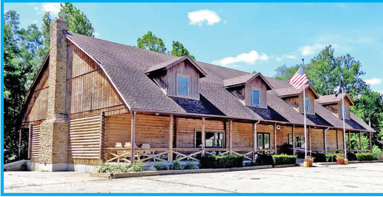
Pendleton American Legion log cabin to receive face lift. (Photo by Rich Creason)
