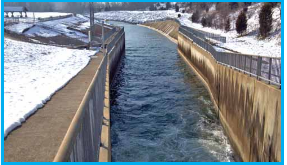
Best place to fish in winter, Stilling Basin at base of Brookville Dam. (Author Photo)
