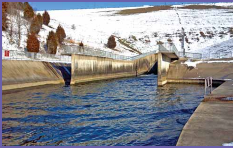
The Brookville Dam Stilling Basin. (Author Photo)
