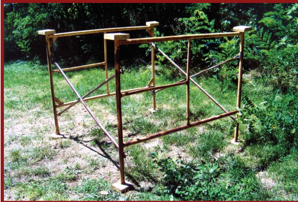
Picture #1: The base construction scaffolding measures 5' x 5' on the ground, with 6" x 6" blocks in place. (Author Photo)
