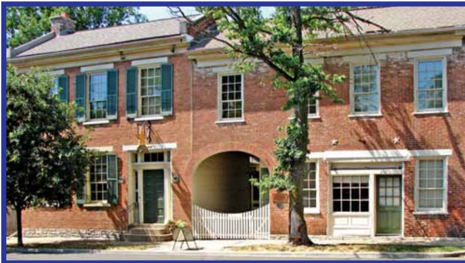
Lantz Archway (1) located at 212 West Main St., c. 1823
