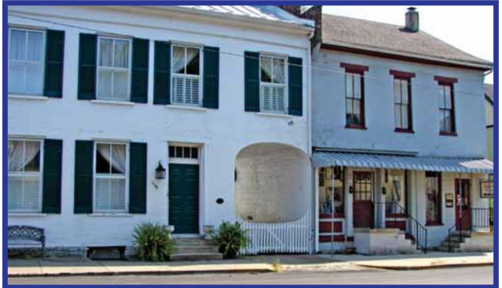
Malone Archway (3) located at 11 West Main St., c. 1836
