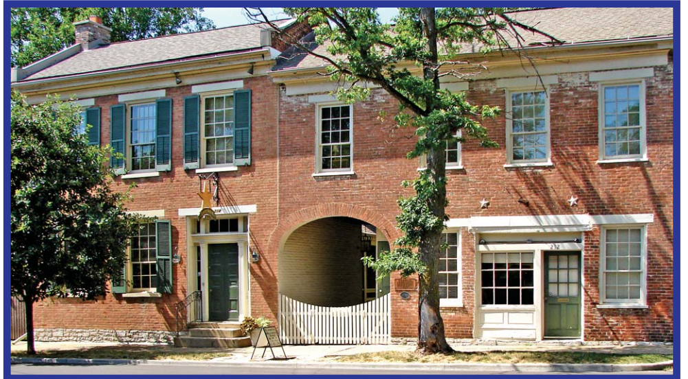
Lantz Archway (1) located at 212 West Main St., c. 1823
