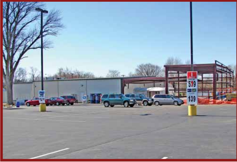
Woodruff's Supermarket at 10 South Main St. in Liberty, Indiana is adding on a 7200 Square addition to their store. Tim Woodruff, owner, is looking to the future with confidence. Tim has always been a leader in his community. (Photo by Ray Dickerson)
