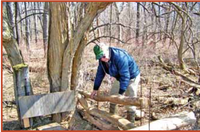
Photo #2 Stacking the logs held in place by old fence posts and rebar. (Photo by Gene Clifford)
