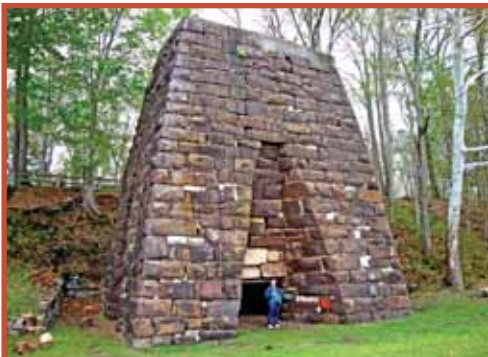
Cornwall Furnace, a cold blast furnace, provided pig iron to the ironworks for the confederates in the Civil War. This is one of the best preserved furnaces in the southeast. (Photo by Susie Creason.)
