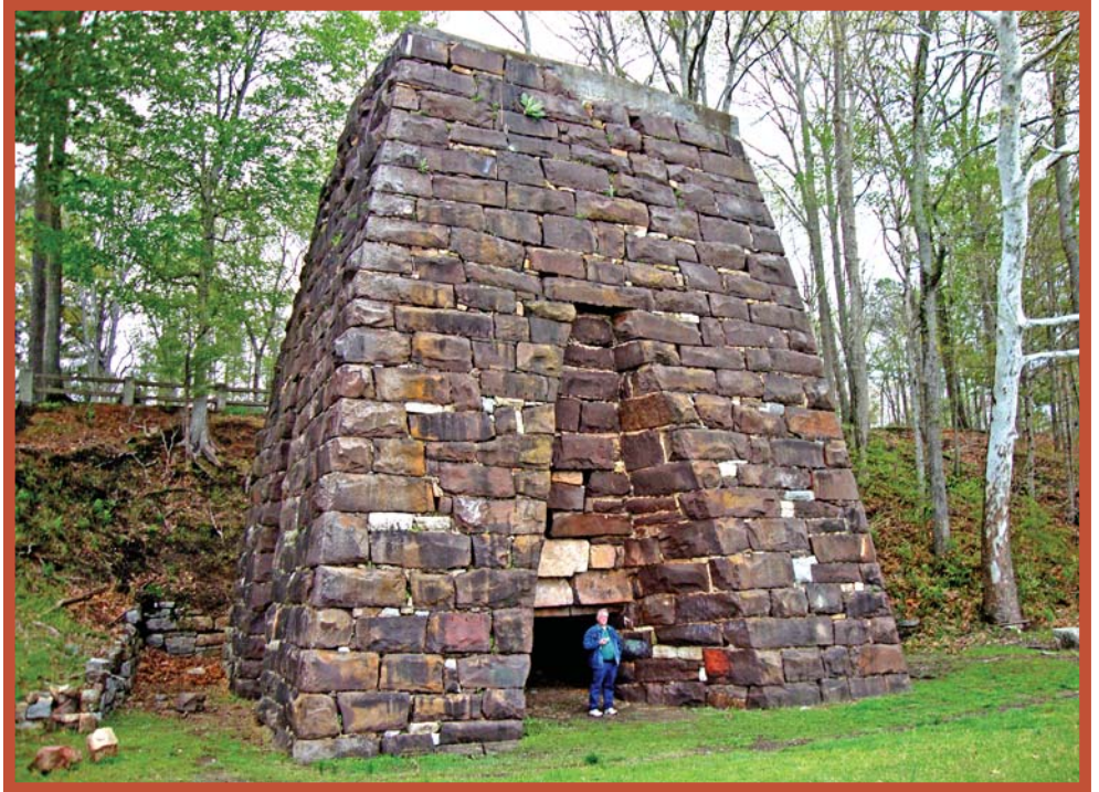
Cornwall Furnace, a cold blast furnace, provided pig iron to the ironworks for the confederates in the Civil War. This is one of the best preserved furnaces in the southeast. (Photo by Susie Creason.)
