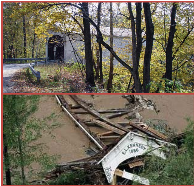
Top: The Moscow Covered Bridge as it looked prior to the 2008 tornado. (Photo by Galen R. Frysinger) Bottom: The Moscow Bridge shortly after the tornado hit. (Channel 8 News Photo)
