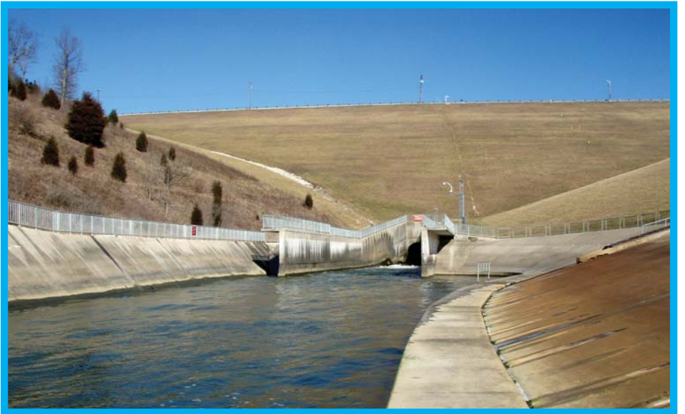
This photo was taken just south of the Stilling Basin. This is where the water comes through the dam from the bottom of the lake. (Photo by Tag Nobbe)
