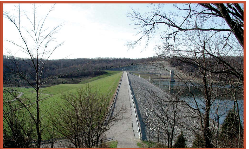
The completed Brookville Lake Dam, this picture taken November 9, 2004. (Photo by Ray Dickerson)
