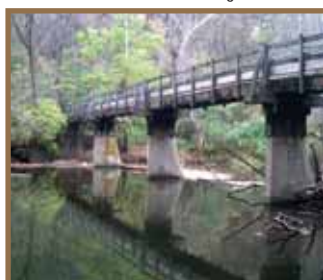
Clifton Gorge Bridge over Little Miami River.
